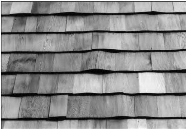
Figure 7. Buckling of shingles installed with insufficient gap.
