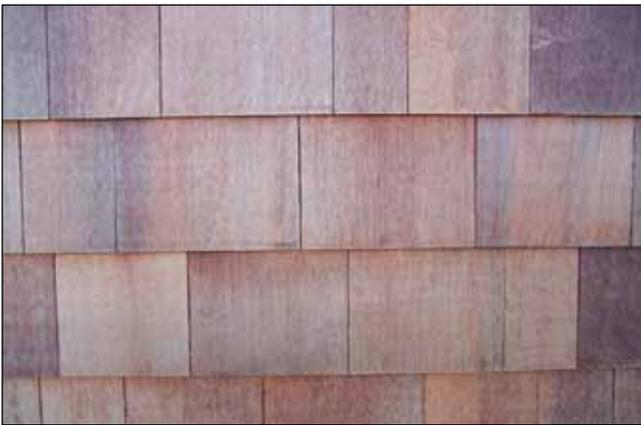
**Figure 13. Shingles treated with tinted water-repellent preservative.**
