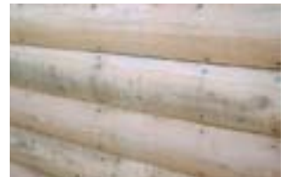
Dark colored streaks from metallic tannates. Oxcon solution will remove rust stains caused by nails, screws and fasteners.
