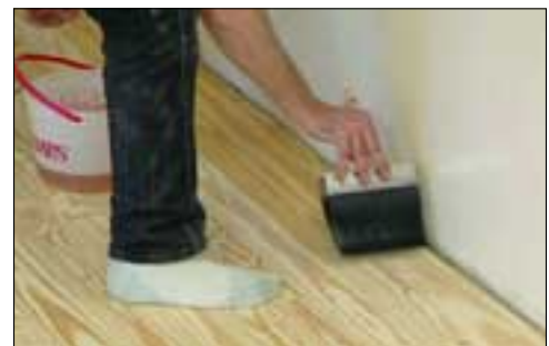
When using a brush, maintain a wet edge, feathering overlaps. Buffing will correct minor errors.
