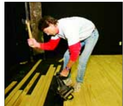
Lengths of flooring are arranged randomly. Using a power nailer, the tongue is blind-nailed to the subfloor nailing base.
