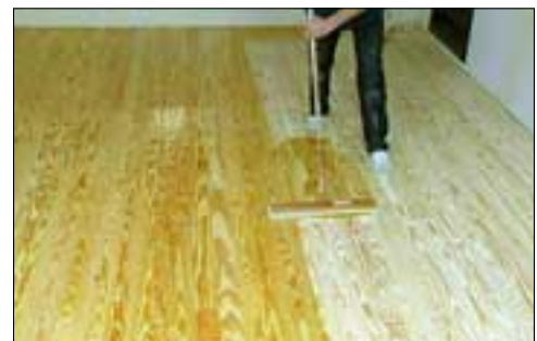
A finish is applied in the same direction as the flooring, using a lambswool pad. New runs overlap about 3”.
