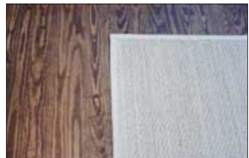
Darker color finishes tend to conceal minor scratches and gouges better than lighter colors, and are well-suited for commercial applications.
