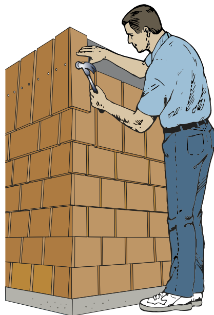
Figure 9: Fitting Laced Corner Courses
